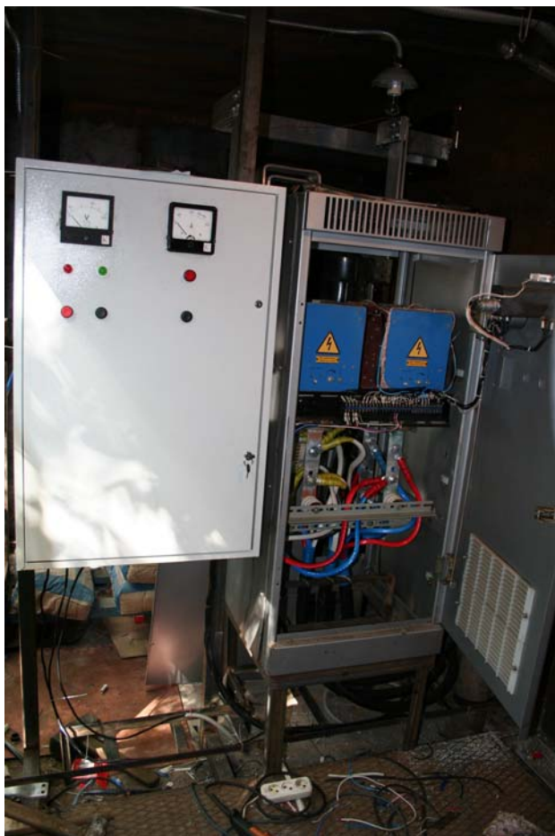
Fig. 3.1.4 - The power transformers installed in the housing and arrangements for their control
