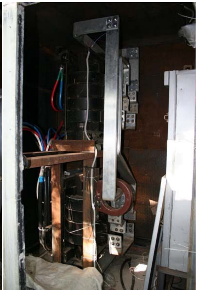
Fig. 3.1.4 - The power transformers installed in the housing and arrangements for their control
