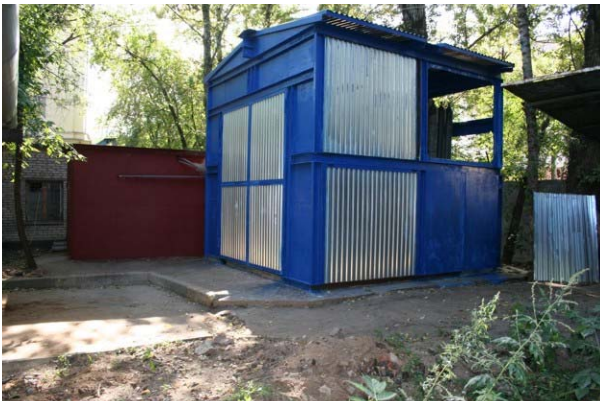
Fig. 3.1.2 - the protective casing and auxiliary housing of the test facility
