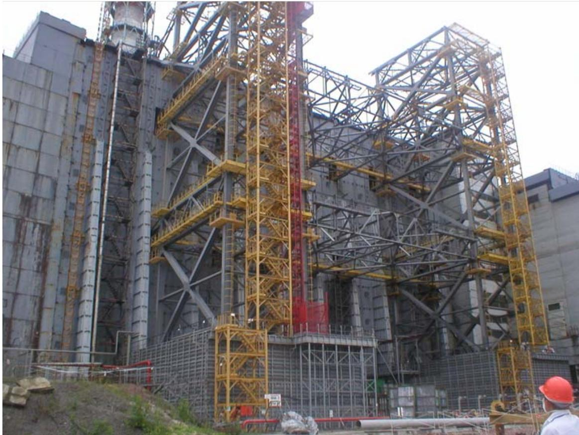
**Figure 3 - Actual view of protective edifice - «Shelter» object after performed works for western fragment stabilization**
