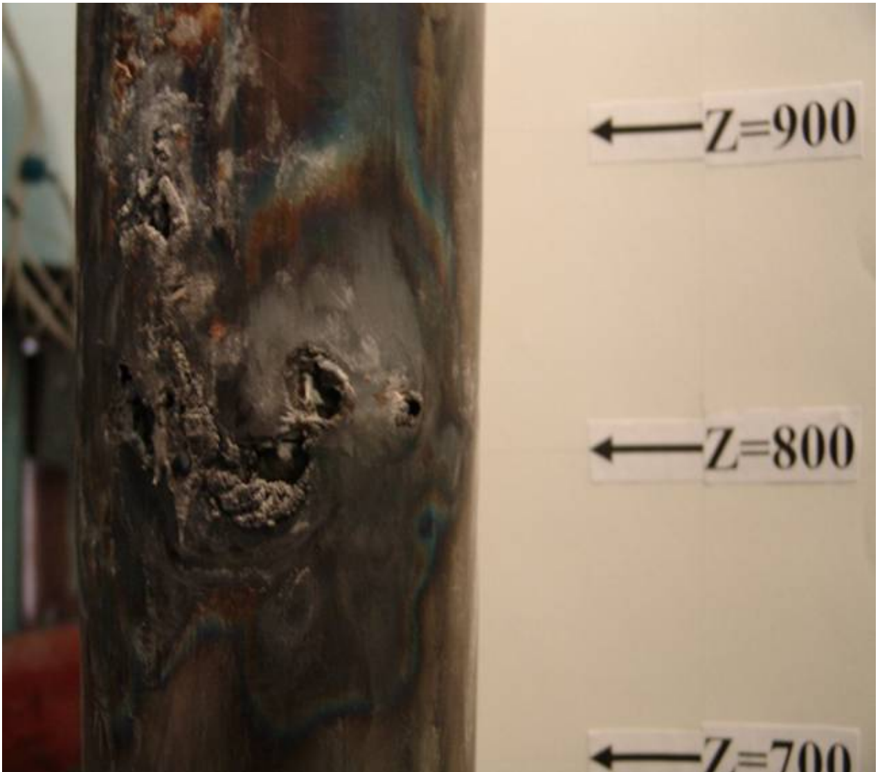
Fig. 21. View of thermoinsulation shroud on the outside at the level of 700 – 900 mm after the experiment.
