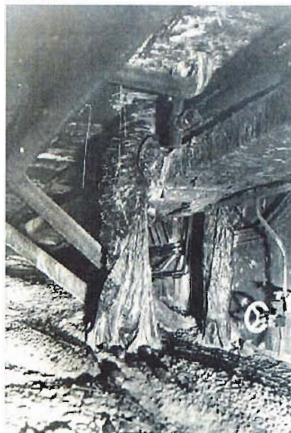
Figure 5.9. – Room #217/2. “Elephant’s foot” and a “Stalactite”
