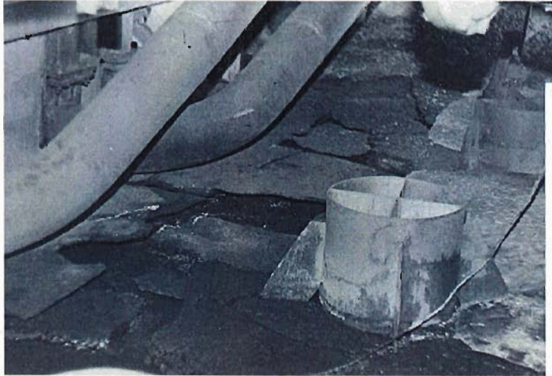
Fig. 5.26. Solidified metal on the floor of Room #210/5
