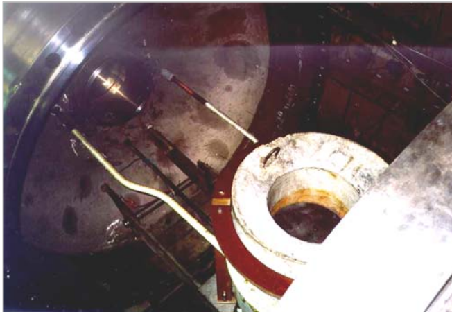
CONCRETE TRAP AND INDUCTION HEATER LOCATED IN MR AND PREPARED FOR CALIBRATION TESTS
