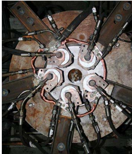
g) Installation of electric wires and water delivery pipelines on plasmatron cooling and gas supply in the inter-electrode space
